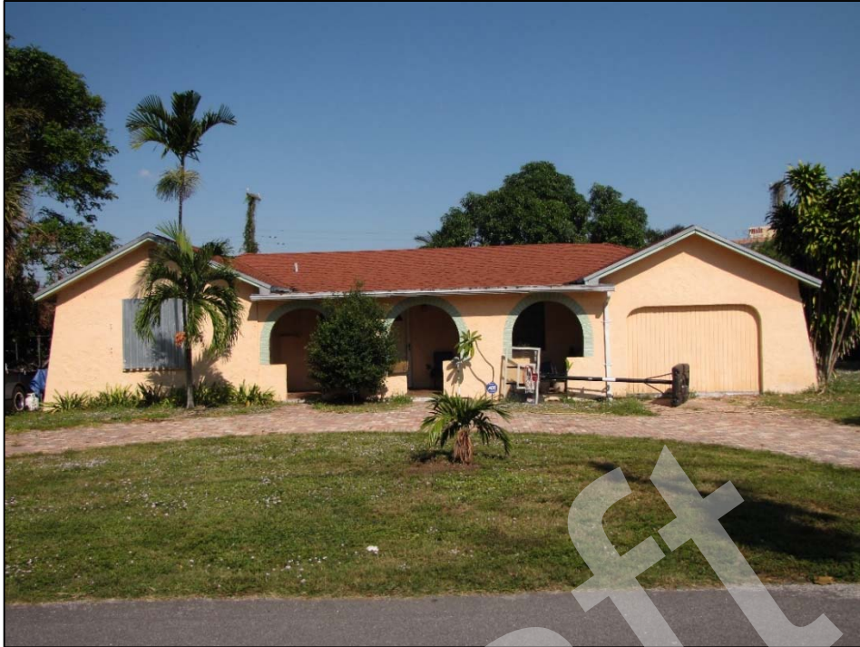
Figure 9.2.87: Newly Recorded 103 Shannondale Road (8PB16468), facing North
