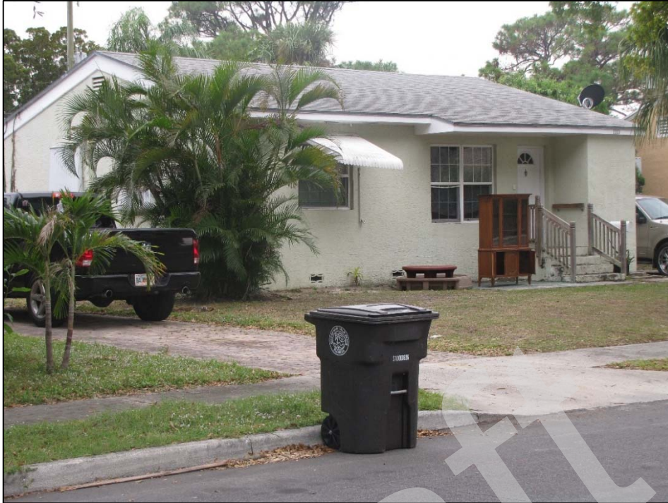
Figure 9.2.67: Previously Recorded 1110 Oak Street (8PB14102), facing Southwest
