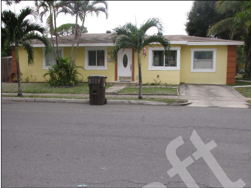
Figure 9.2.43: Previously Recorded 3801 Merrill Avenue (8PB14065), facing West
