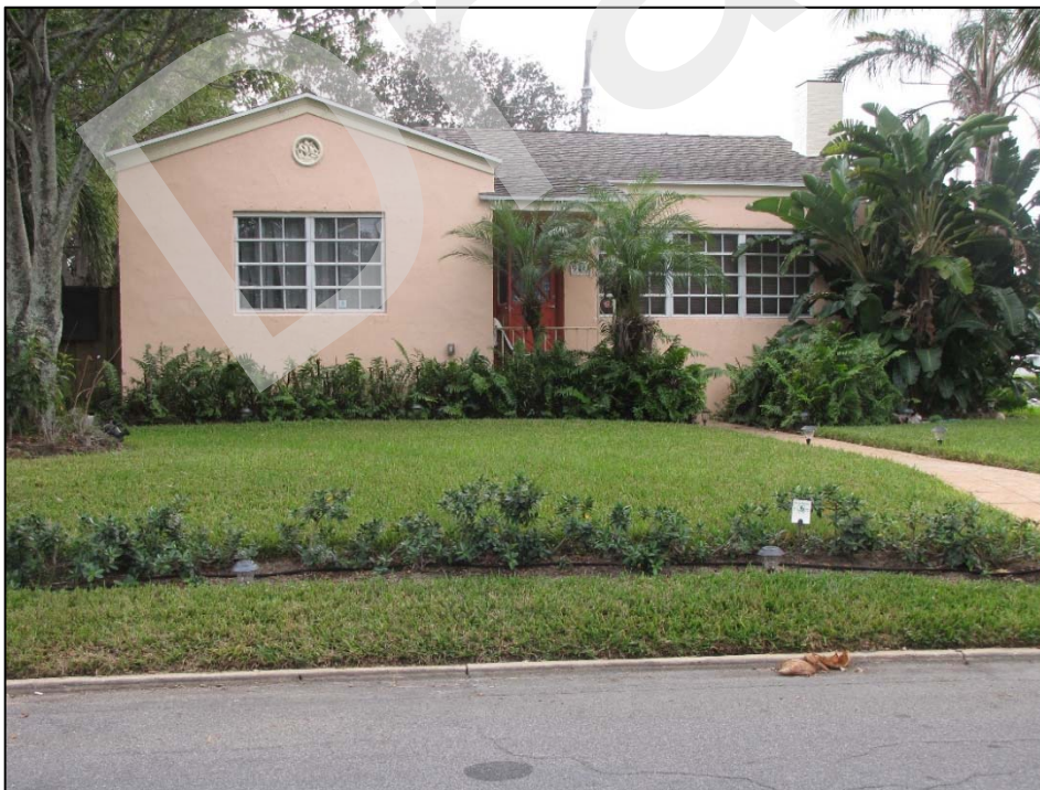
Figure 9.2.22: Previously Recorded 946 Paseo Andorra (8PB13970), determined a contributing resource to the Vedado Historic District (8PB14206), facing South
