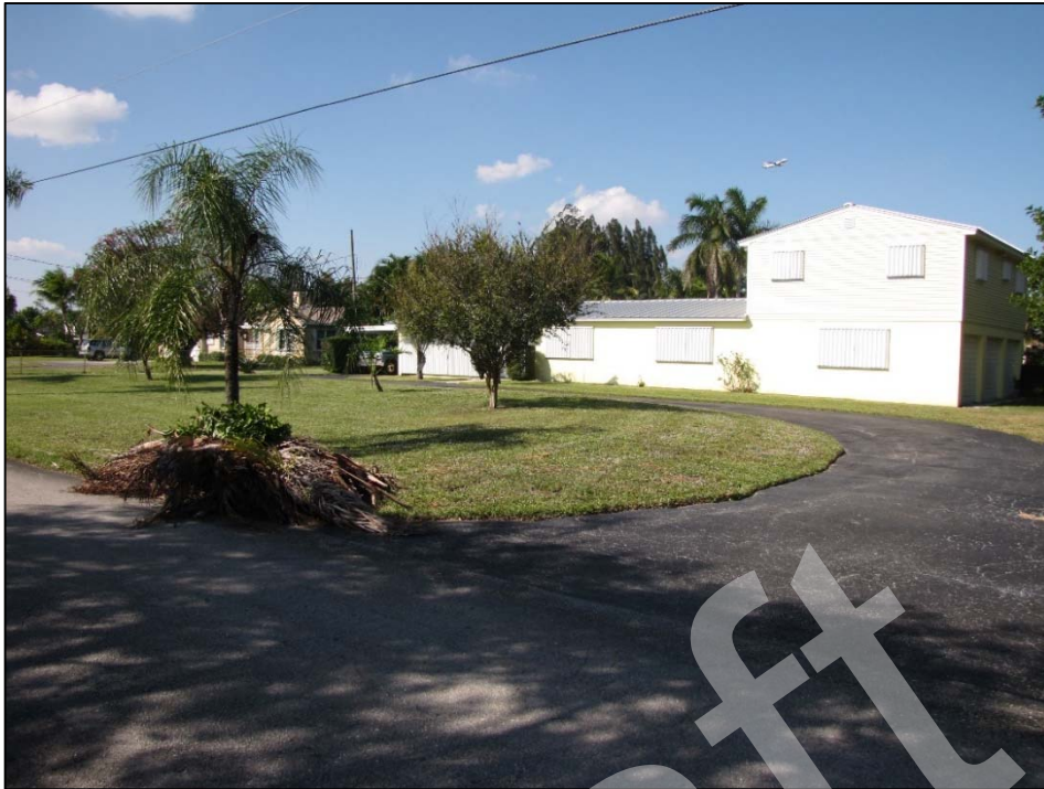
Figure 9.2.13: A Streetscape at the North side of Churchill Road in the Town of Glen Ridge, facing Northwest
