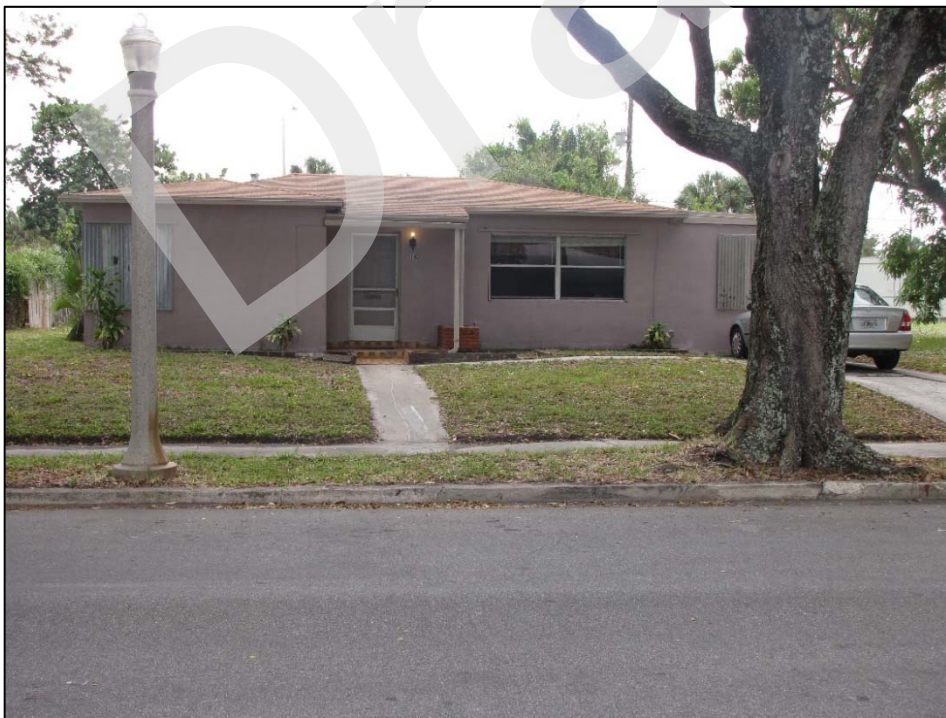
Figure 9.2.54: Previously Recorded 1110 Van De Venter Street (8PB14088), facing South
