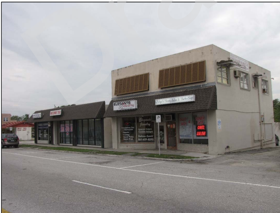
Figure 9.2.102: Newly Recorded 4121 Parker Avenue (8PB16483), facing Southwest
