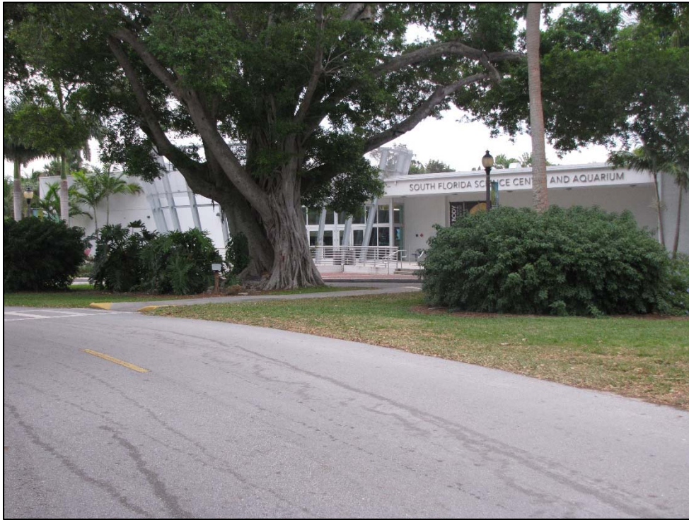
Figure 3: The 1971 and 2014 Additions to the South Florida Science Museum, facing Southeast
