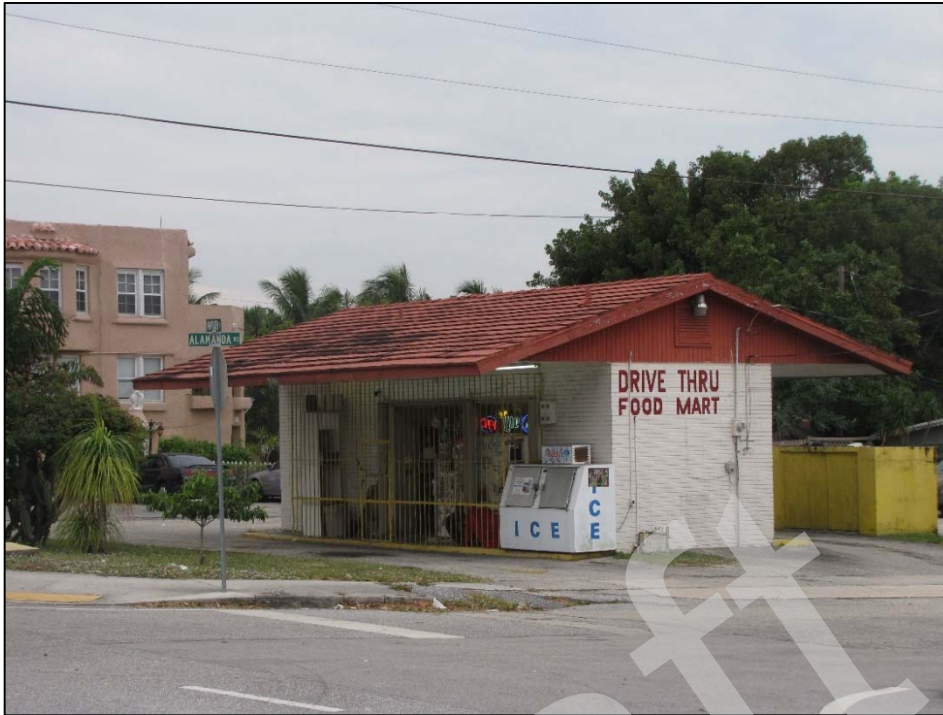
Figure 9.2.103: Newly Recorded 4201 Parker Avenue (8PB16484), facing Southwest
