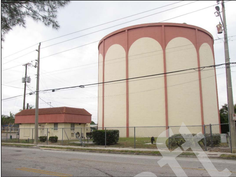
Figure 9.2.105: Water Tower / 4400 Parker Avenue (8PB16486), facing Northeast
