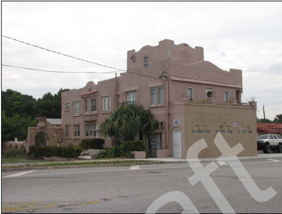
Figure 9.2.29: Previously Recorded 4211 Parker Avenue (8PB3588), facing Northwest
