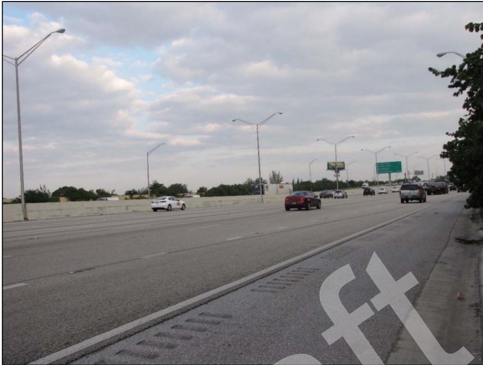
Figure 9.1.4: I-95 North-bound Lanes from the Southern End of the APE, facing Northwest
